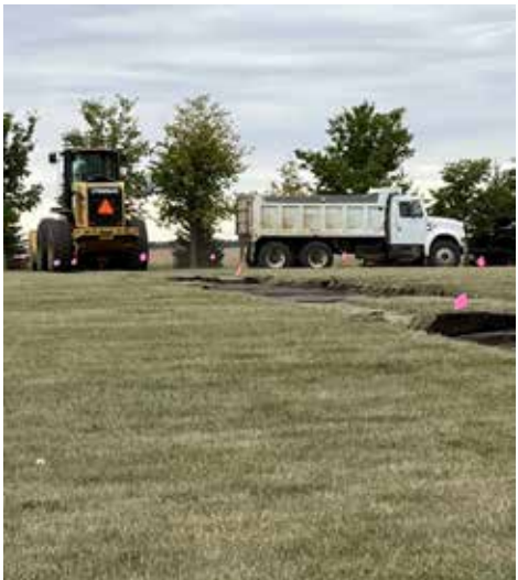
Some of the construction vehicles used to cut the new roads through the De Smet Cemetery. (Photo by Sheryl Downes)
