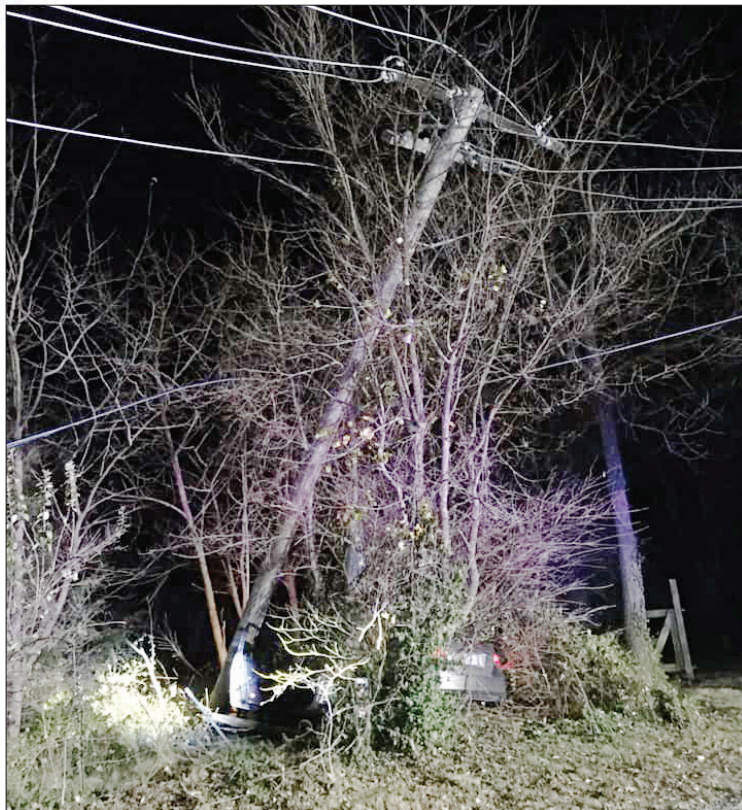
Photo courtesy of the City of Lebanon A car crashed into an electric pole Wednesday night in the area of Wood and Cherry streets, causing a power outage.
