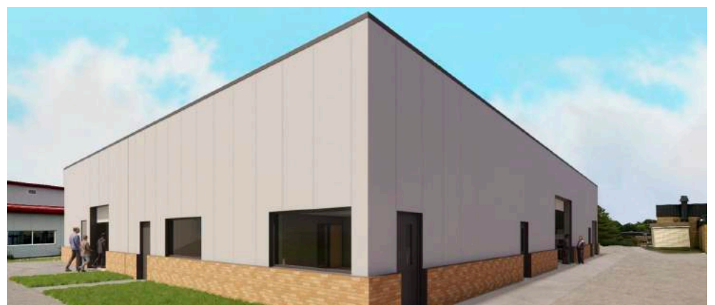
Work on remodeling the welding and metals lab should begin in March.
