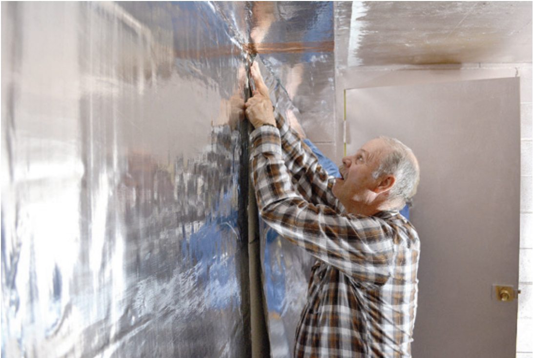
Working in the basement of the Park County Office Building last week, outgoing Park County Homeland Security Coordinator Mart Knapp smooths out some foil that’s meant to shield the room from electromagnetic pulses (EMPs) or solar flares that can destroy electronic devices. Tribune photo by CJ Baker
