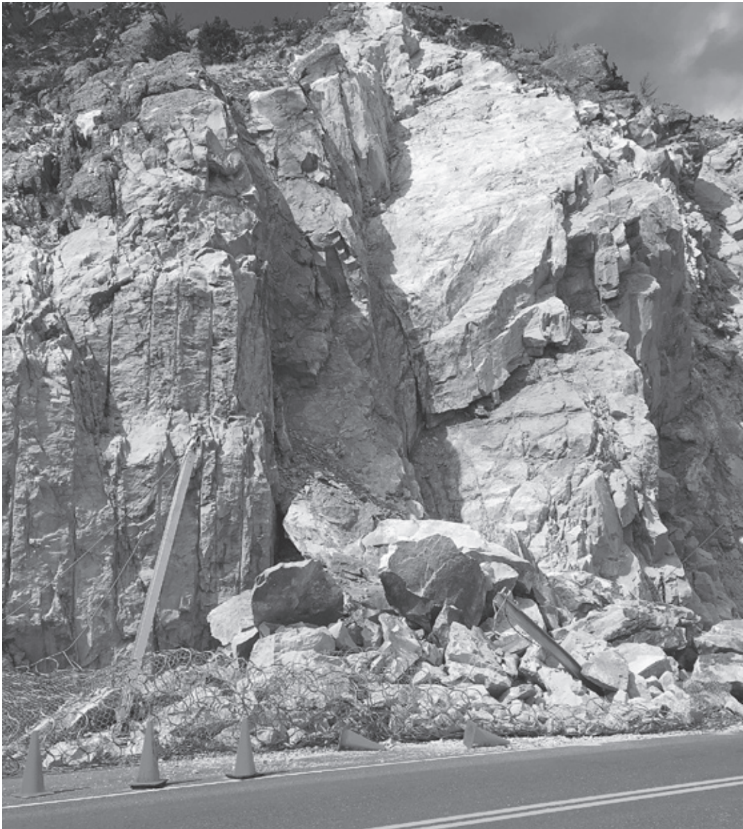
Like a big catcher's mitt, the mesh wire fence 'snagged' sliding rocks off the mountain above U.S. Highway 14/16/20, near Buffalo Bill Dam. WYDOT will repair the fence damaged by the Memorial Day weekend slide. Tribune photo by Dave Bonner
