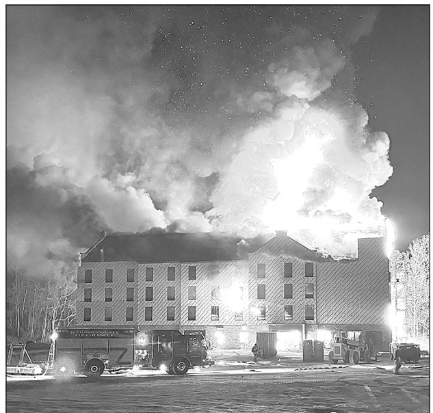
Savannah's newest hotel, the Sleep Inn, was under construction before being destroyed by a suspected arson fire on December 11, 2024. Photo from Hardin County Fire Department.
