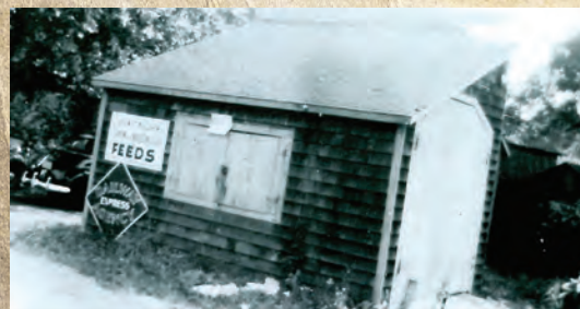
Nitrate/Soda Storage Building
