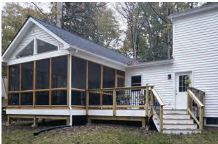
Exterior and Porch Renovations
